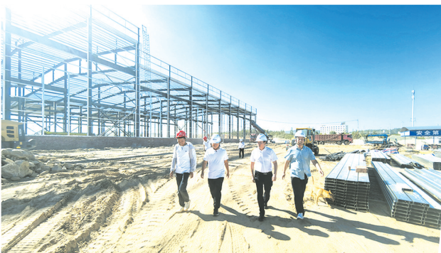
▲ 钾长石科技产业园建设现场
